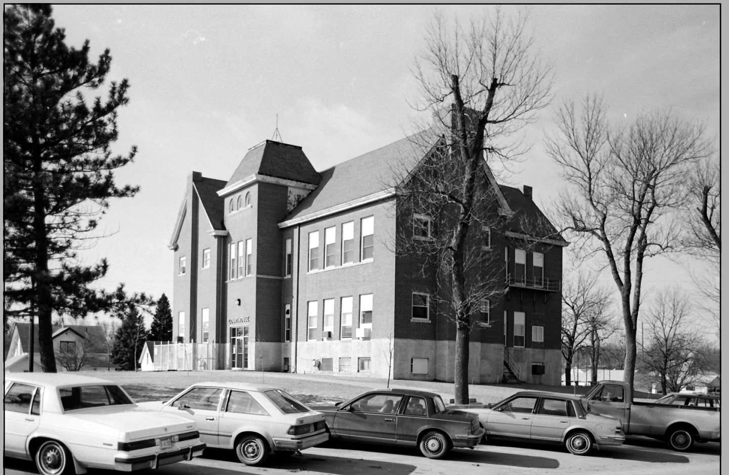
View looking southwest showing north and east facades. Photo by BJB Long, Four Mile Research, 1989, NSHS (8903/5:31)
