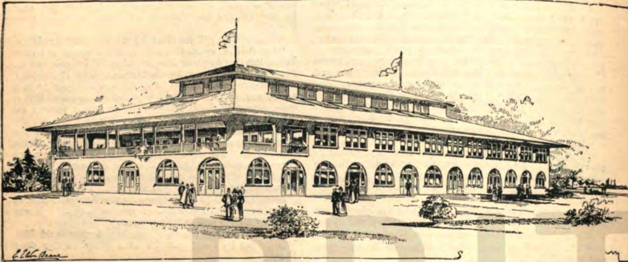
THE DAIRY BUILDING.
