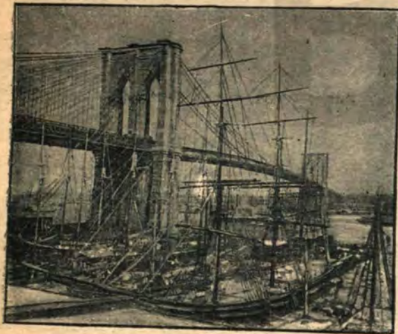
BROOKLYN SUSPENSION BRIDGE.
