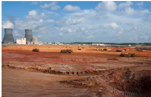
Construction site of new units at Plant Vogtle
