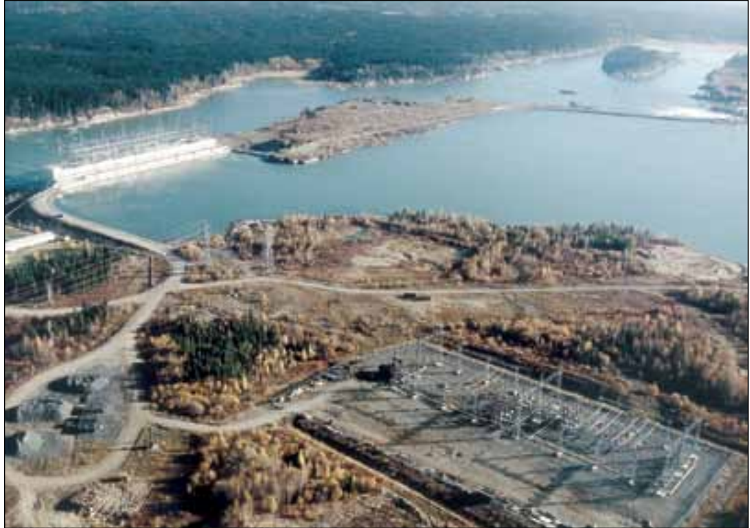
This aerial view of Kelsey Generating Station shows the powerhouse (upper left) and the spillway (far upper right) a short distance away. The geography of the area did not lend itself well to having the spillway built "run-of-river" — that is, built adjacent to the powerhouse.
