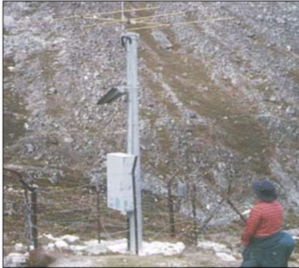
Figure 5.6: Installation of early warning system (Source: http://hmg.npolar.no/opencms/export/sites/hmg/en/documents/topic-2/reynolds2_topic2.pdf )
