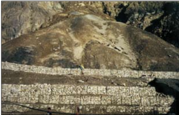
Figure 10.9: Gabion wall constructed to stabilize uphill slope 12
