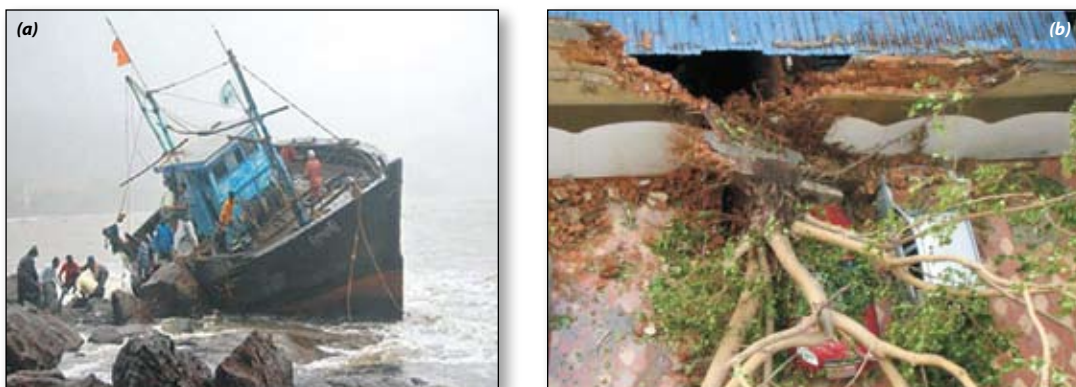
Figure 2.17 . a : Damages caused by the cyclone 'Phyan' in the coastal parts of Maharashtra and Goa, India (Source: http://www.imd.gov.in/section/nhac/dynamic/rsmc.pdf ). b. Destruction caused due to cyclone Phyan (Source: http://www.zimbio.com/Tropical+cyclones/articles/123UgglbFBo/Mumbai+Rains+Today+Mumbai+Cyclone+Mumbai+Weather )
