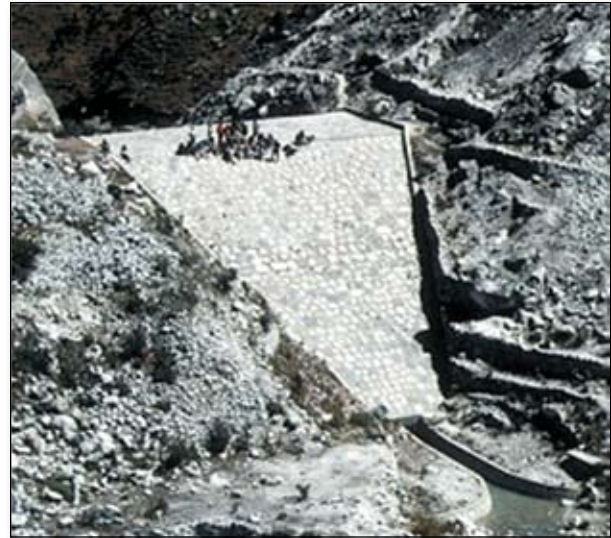
Figure 5.7: Channel and moraine dam built in reducing impact of GLOFs. (Source: http://hmg.npolar.no/opencms/export/sites/hmg/en/documents/topic-2/reynolds2_topic2.pdf )
