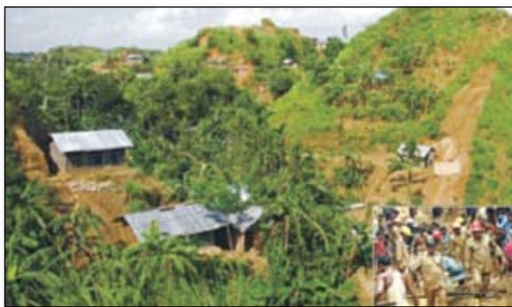
Figure 10.5: Houses built by cutting hills at Salimpur area of Chittagong city hoodwinking consequence. Inset, firemen and locals recovering a body at Harinmara of Lama in Bandarban after the mudslide (Source: Star)
