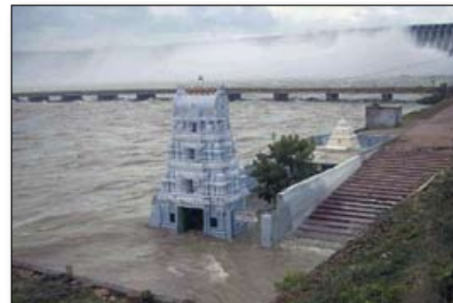
Figure 3.17: A swollen Krishna River flowing a few feet below the railway track downstream of the Prakasam Barrage in Vijayawada, Andhra Pradesh. (source: whatslatest.com)
