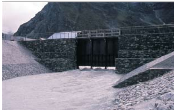
Figure 5.8: Channel for creating outlet from glacial lakes (Source: http://hmg.npolar.no/opencms/export/sites/hmg/en/documents/topic-2/reynolds2_topic2.pdf )
