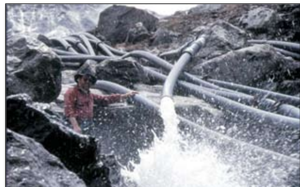
Figure 5.9: Installation of siphons for diverting water from glacial lakes (Source: http://hmg.npolar.no/opencms/export/sites/hmg/en/documents/topic-2/reynolds2_topic2.pdf )
