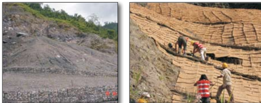
Figure 10.11: Plantation work (left) and application of ROFA (right) 12
