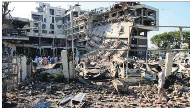
Figure 12.29: Site of bomb blast in the Pearl Continental hotel in Peshawar (Source: BBC News).
