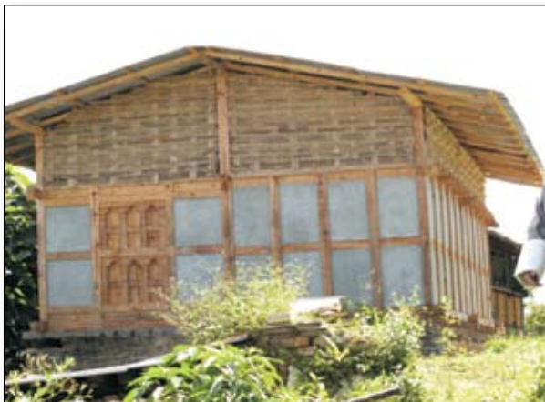
Figure 9.15: Undamaged Ekra structure (Source: SQCA Bhutan)
