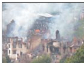
Figure 12.15: The burning remains of a conflagration that gutted 12 houses in Wamrong
