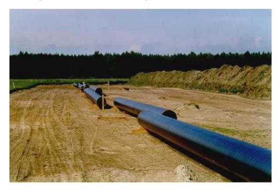
The 22" Onshore Pipeline connects the Mazeikiai Refinery Pumpstation with the Butinge Oil Terminal. The total length is 91,6 km.
