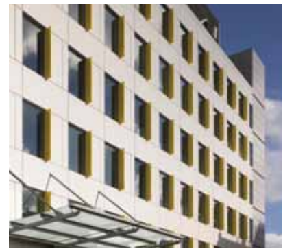
Two views of the L Block development at the Hammersmith Campus, which is nearing completion.
