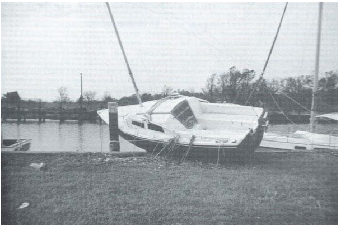
FIGURE 37. Marina Damage at Battery Park, Apalachicola.
