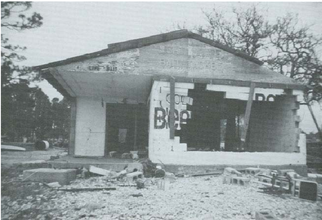
FIGURE 31. Heavy wave damage to another commercial building.
