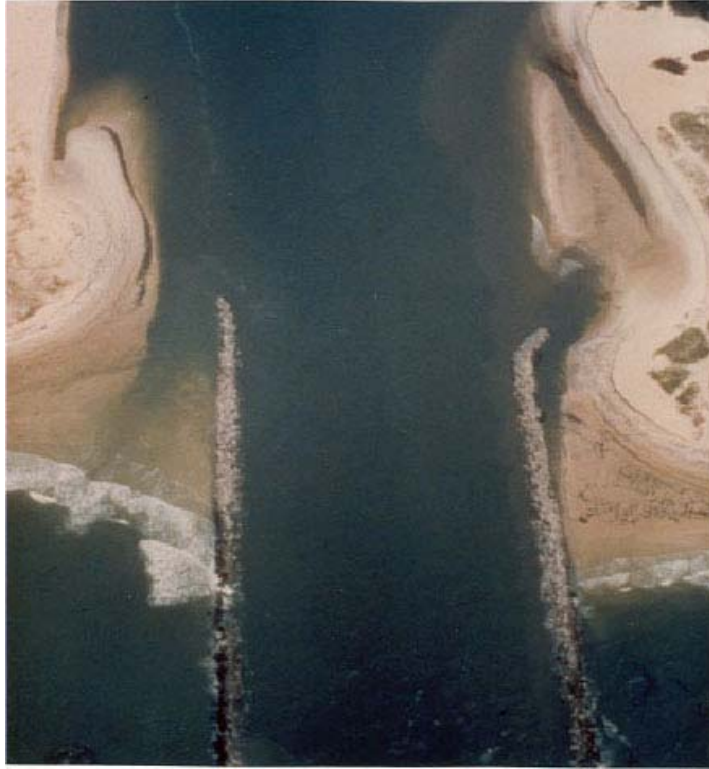
FIGURE 39. Sike's cut (St. George Island Channel) in November, 1985 prior to Kate (photograph by Kevin R. Bodge).
