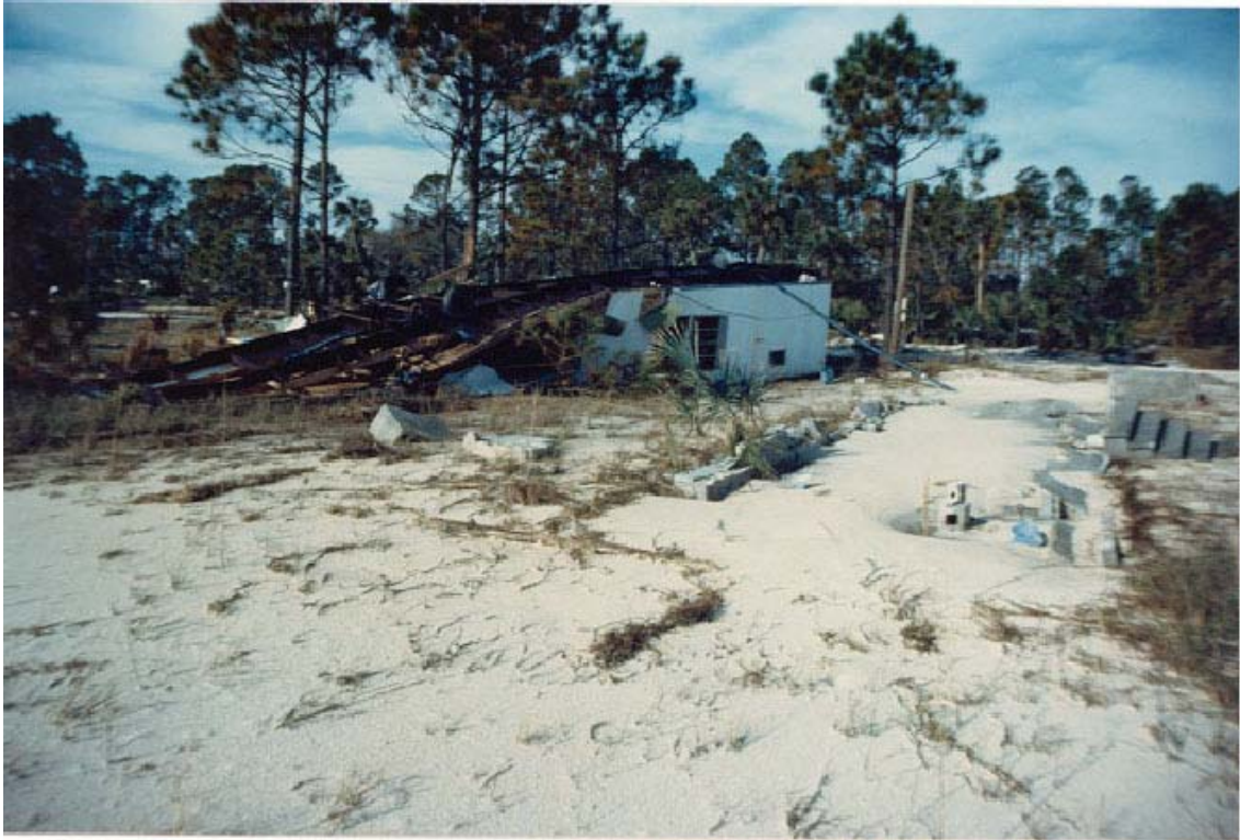
FIGURE 26. Mobile home destroyed by wind and flooding.
