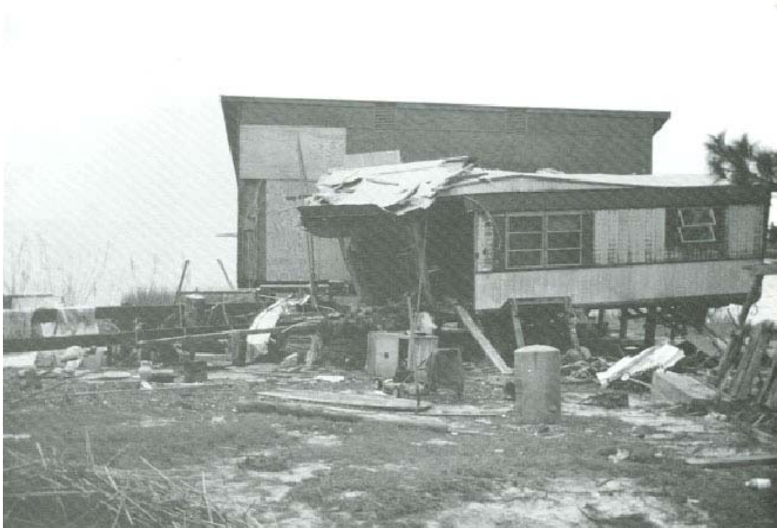
FIGURE 34. Apalachicola Bay shoreline dwelling destroyed.
