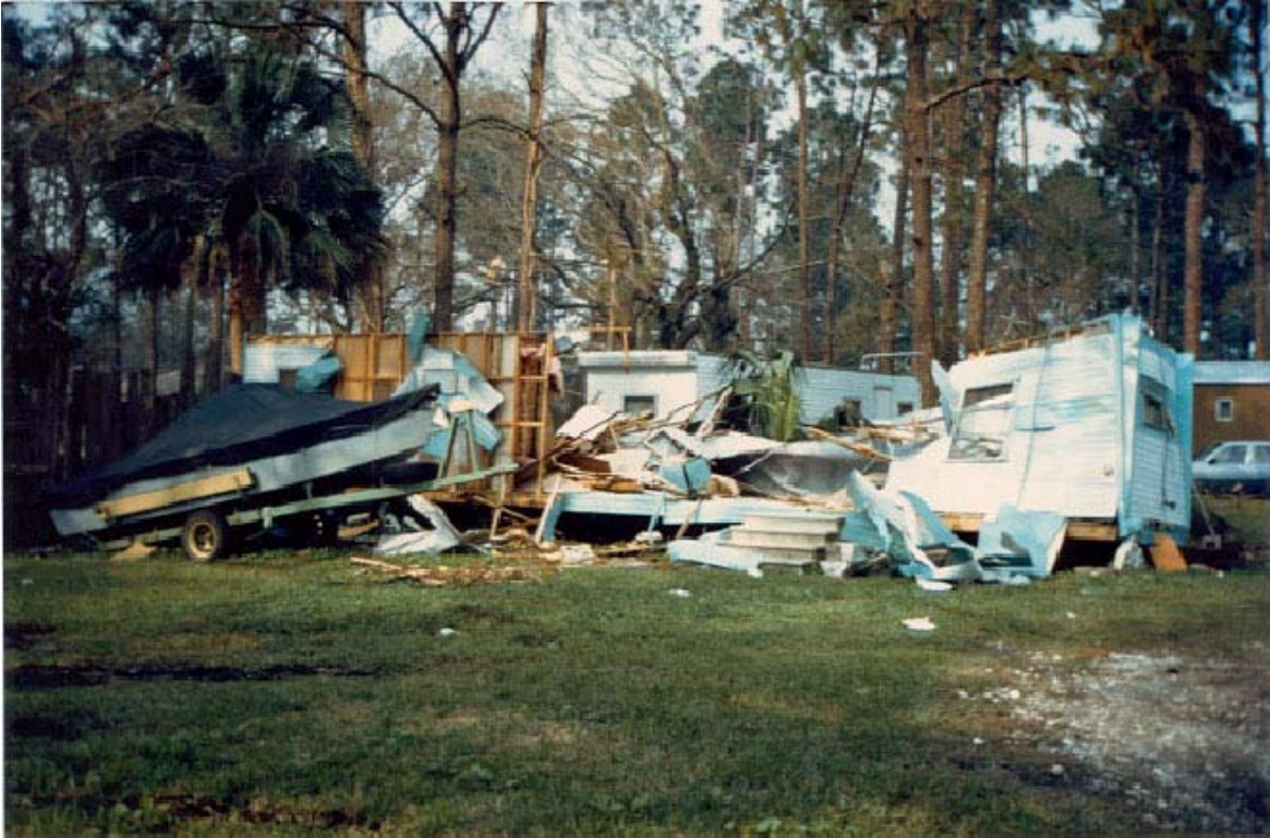
FIGURE 32. Mobile home destroyed by wind.
