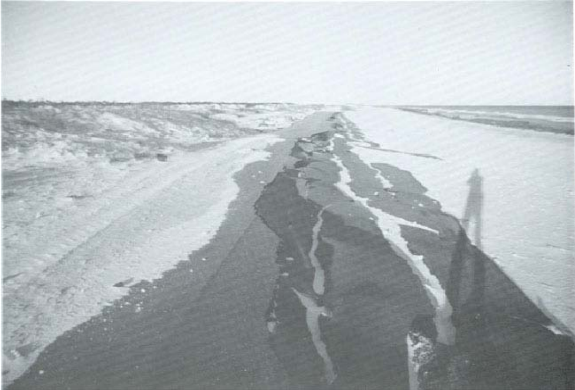
FIGURE 54. St. George Island State park road destroyed.
