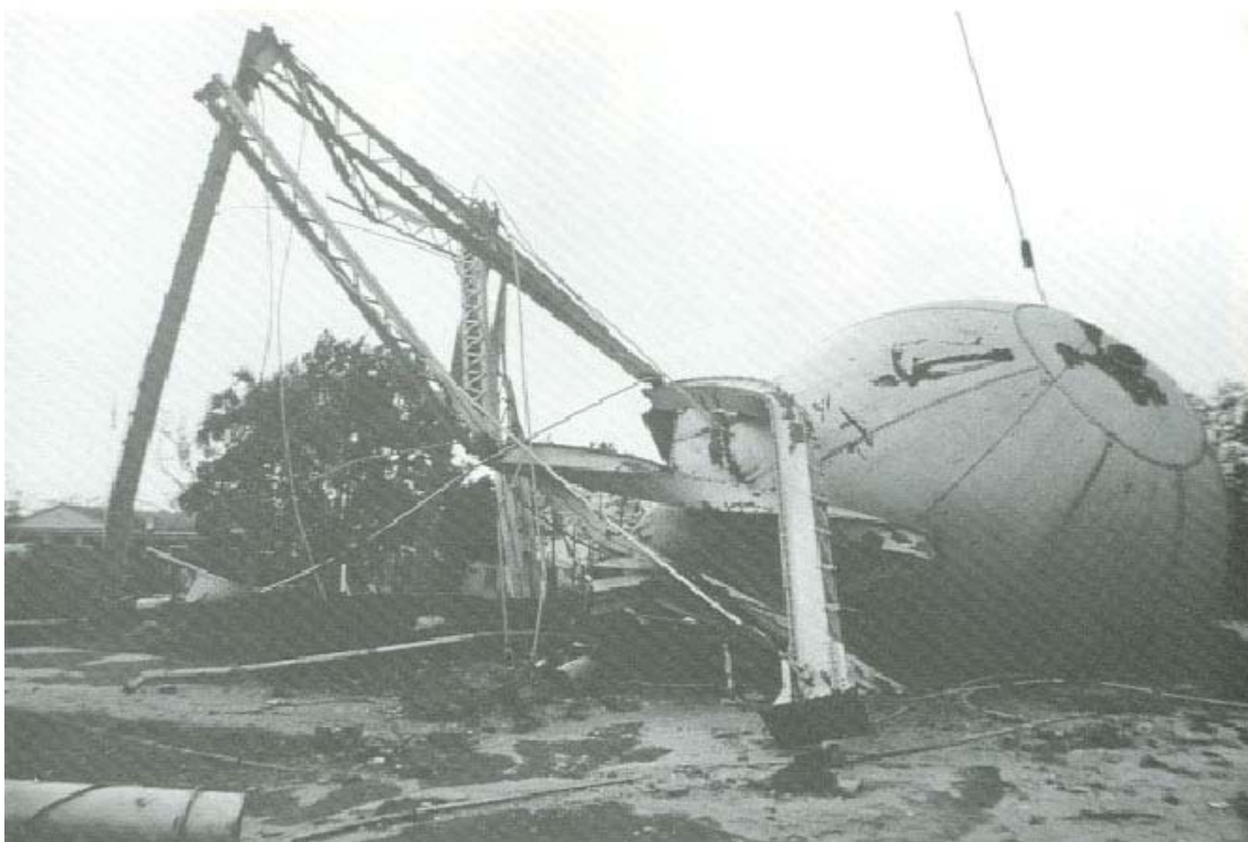
FIGURE 35. One hundred year old Apalachicola water tower toppled by Kate's winds.
