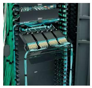
The modularity of preterminated fiber and copper cabling also enables high densities per unit of rack space, which promotes efficient use of valuable data center real estate and makes them suited for deployment throughout the data center.
