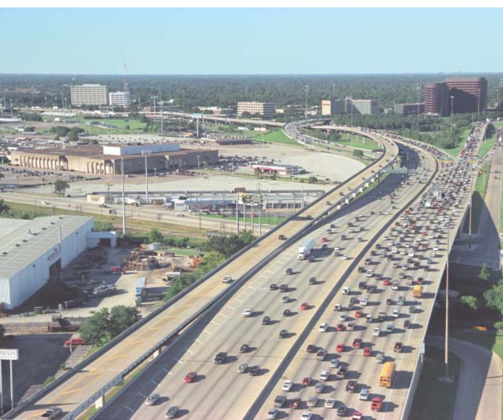
The elevated bypass: Carpools and buses on the two-way elevated transitway structure along the West Loop North zoom past backed-up traffic on the freeway main lanes. (Photo: September 2002)
