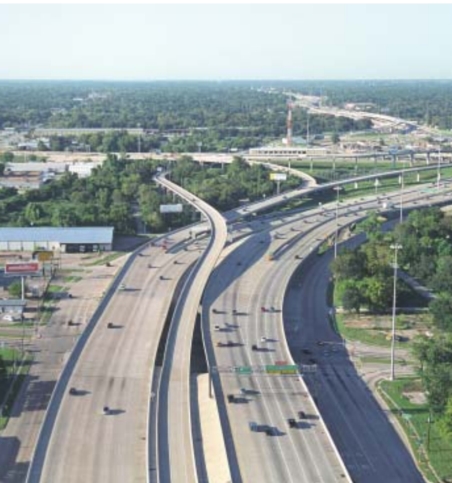
The interchange bypass: Transitways were added to freeways after the original freeway construction, necessitating structures to get around existing interchanges. A long elevated structure allows transitway vehicles to bypass the IH 10-IH 45 interchange north of downtown. The elevated bypass opened on October 16, 2000. (Photo: May 2002)
