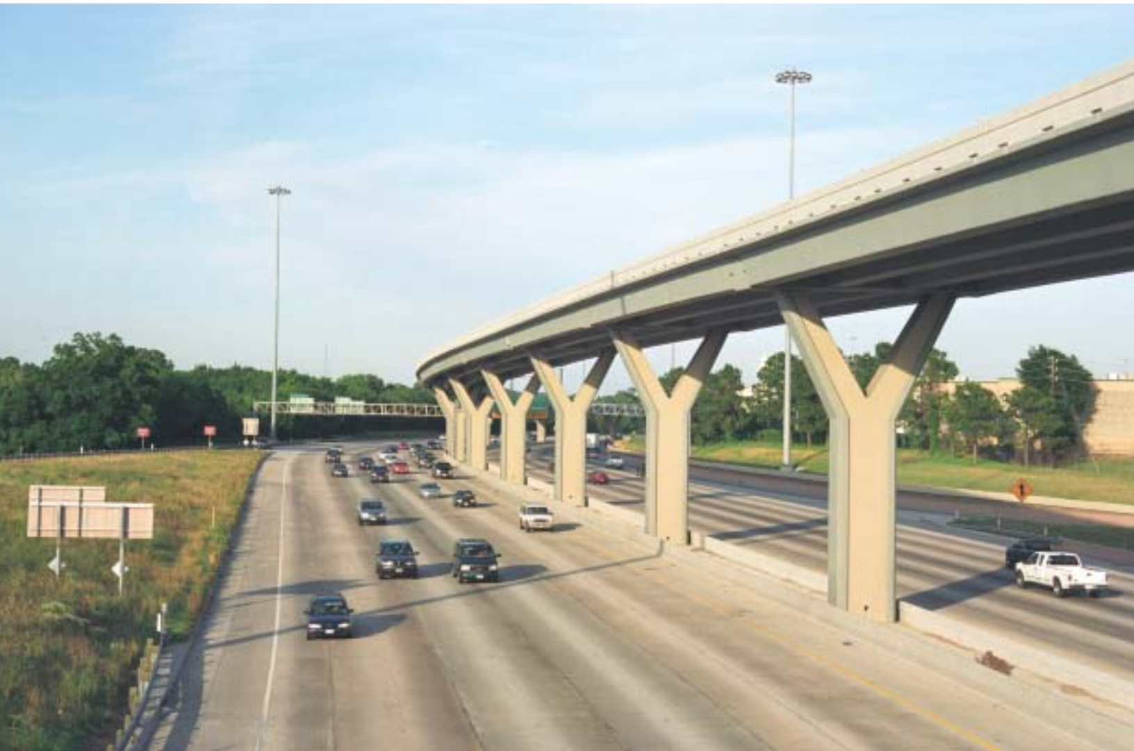
Downtown access ramp: This view shows the elevated structure for the two-way transitway ramp along the downtown approach of the Katy Freeway (IH 10). (Photo: May 2002)
