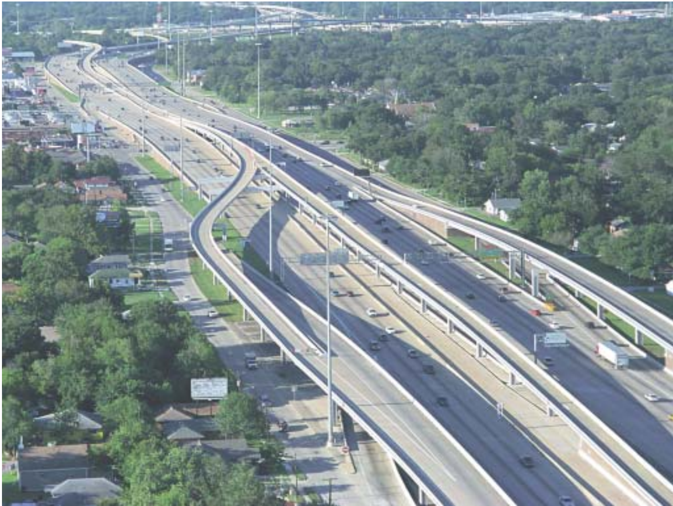
The half-wishbone: This structure on the Eastex Freeway allows southbound transitway vehicles to exit to the freeway main lanes. (Photo: September 2002)
