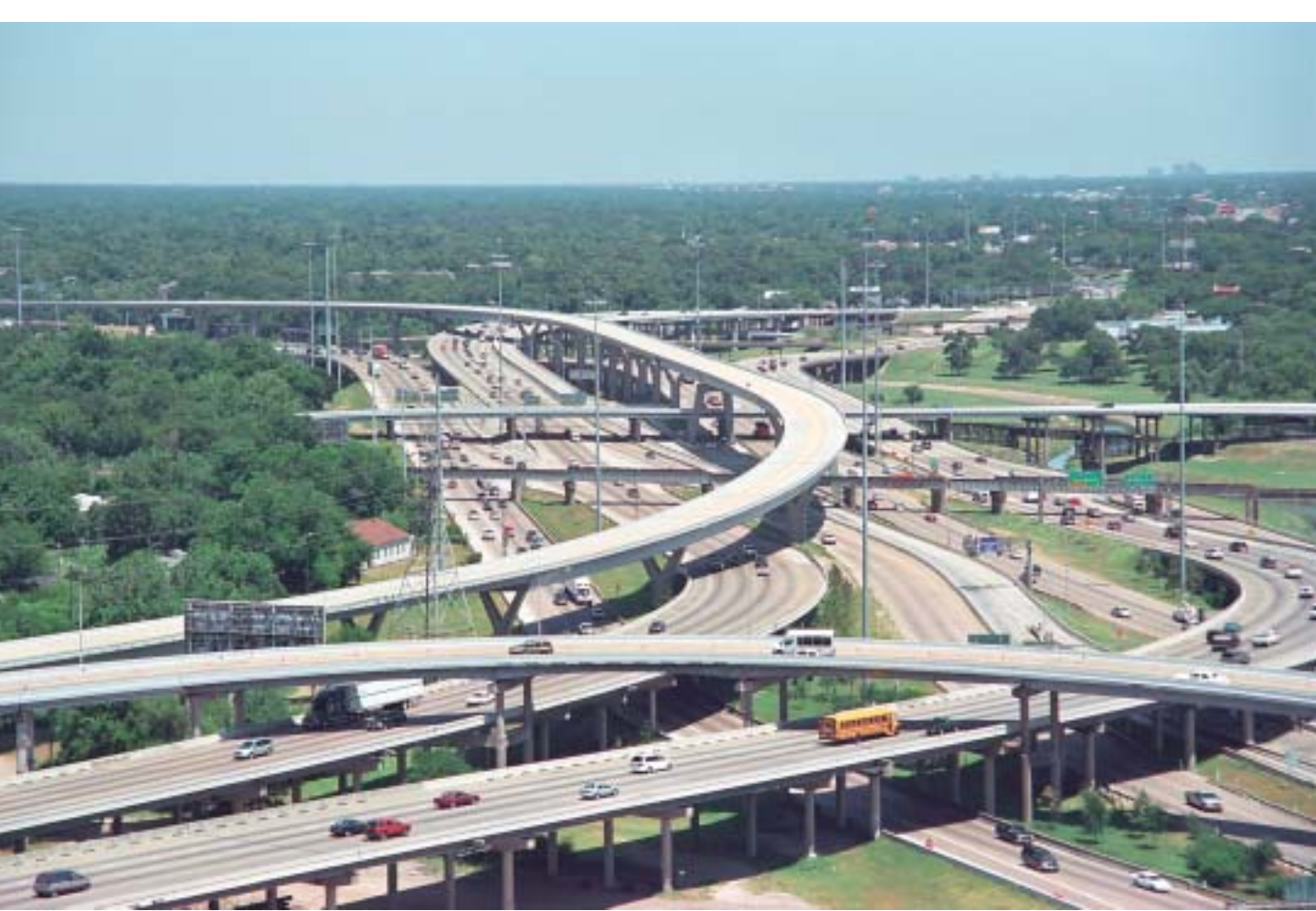
The interchange bypass: Transitways were added to freeways after the original freeway construction, necessitating structures to get around existing interchanges. A long elevated structure allows transitway vehicles to bypass the IH 10-IH 45 interchange north of downtown. The elevated bypass opened on October 16, 2000. (Photo: May 2002)
