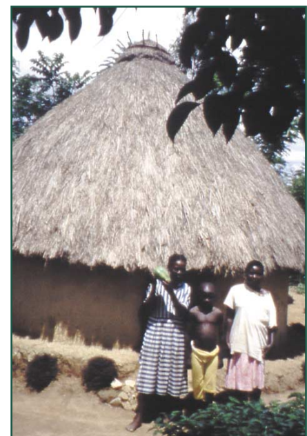
External view of house – West Kenya
