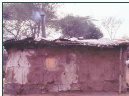
Maasai house, showing window (closed) and smoke coming out of chimney
