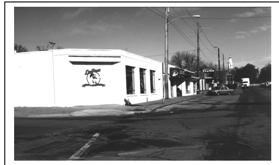
Typical Roofline along Washington Street
