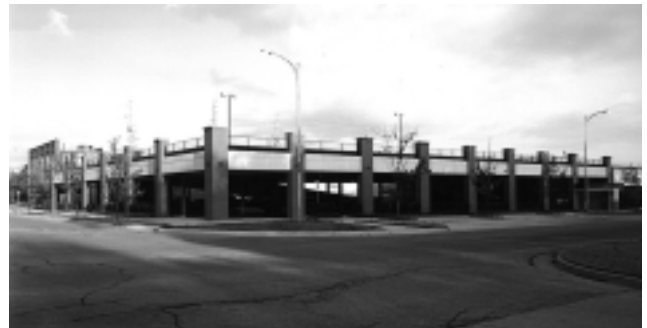
Existing Parking Structure
