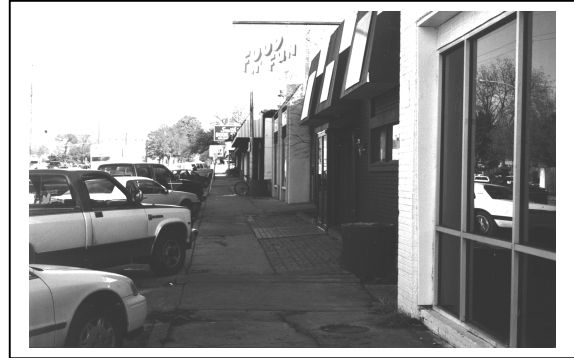
Glass Storefronts along Washington Street
