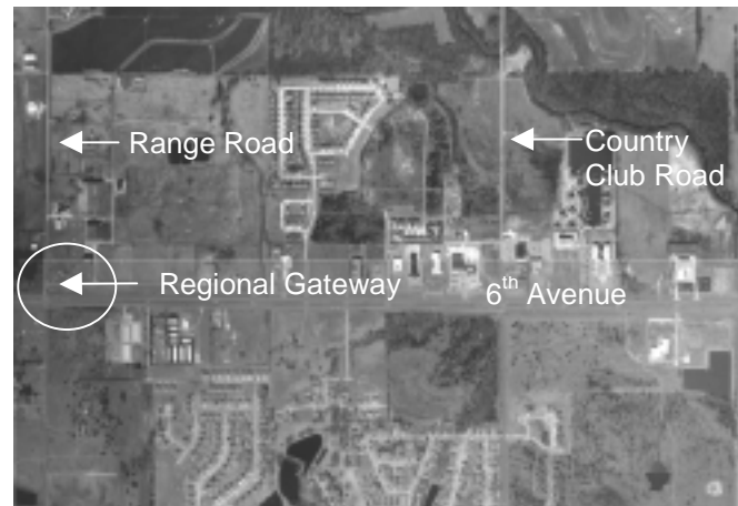
Regional Gateway at Range Road and 6 th Avenue
