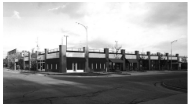
Proposed Phase One Improvements illustrating retail commercial use & fronts on street level
