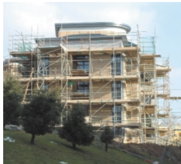
Colman House starts to take shape
