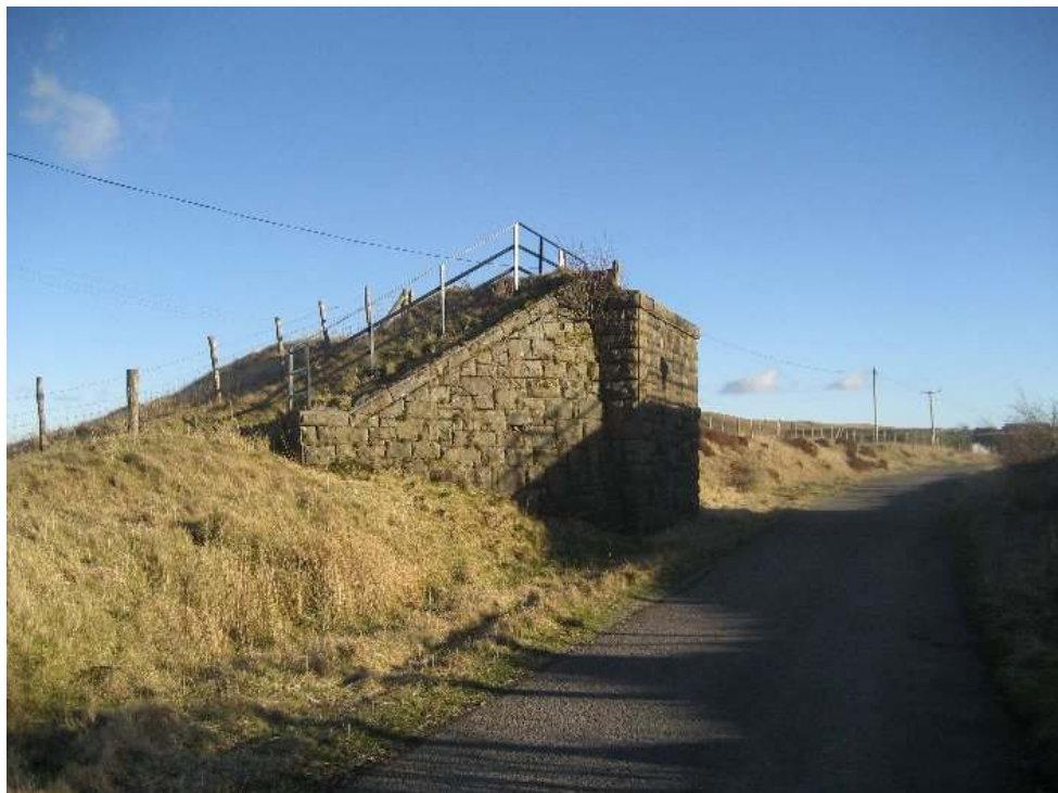
Fig.9 A view south east at the eastern abutment of 'Racehorse Road' bridge, close to Waunavon which once carried a small road to a group of nearby dwellings. Access is now provided by the tarmac road between the abutments on the line of the railway
