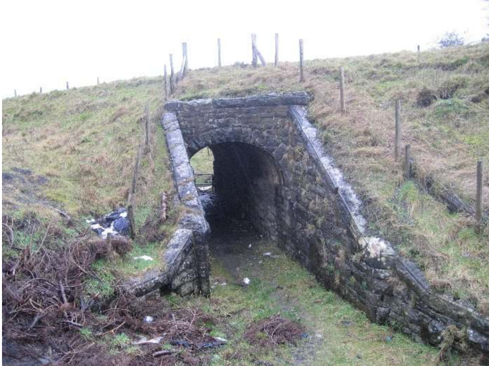
Fig.8 The attractive arch over which the line once ran, and which would be just outside the proposed Brynmawr station. The arch once carried the Nantyglo Level tramway.
