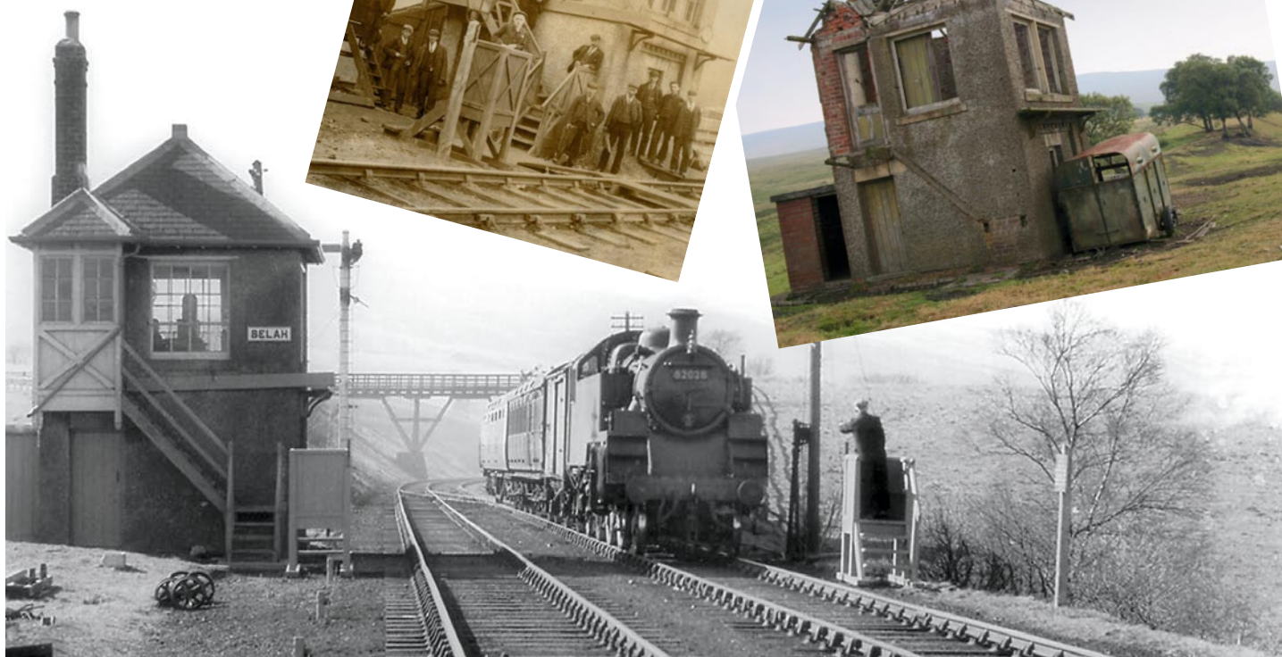
(Above left) Belah signal box and staff circa 1892 and (above right) its sad remains.
