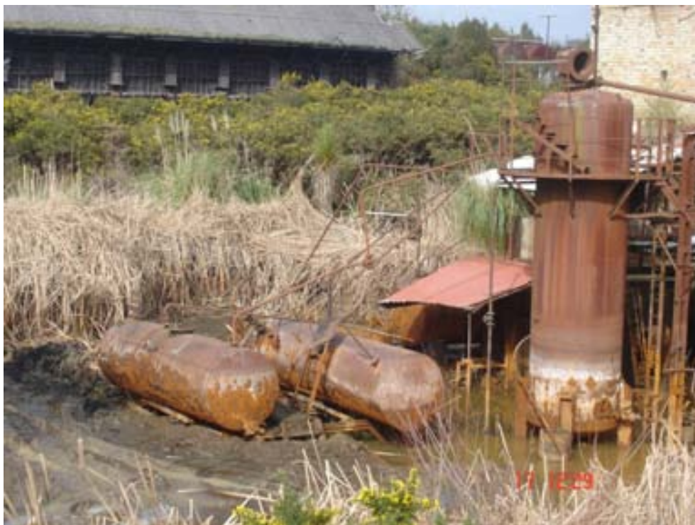
Photo 4: WCP following dewatering, showing existing above ground storage tanks containing residual coal tar
