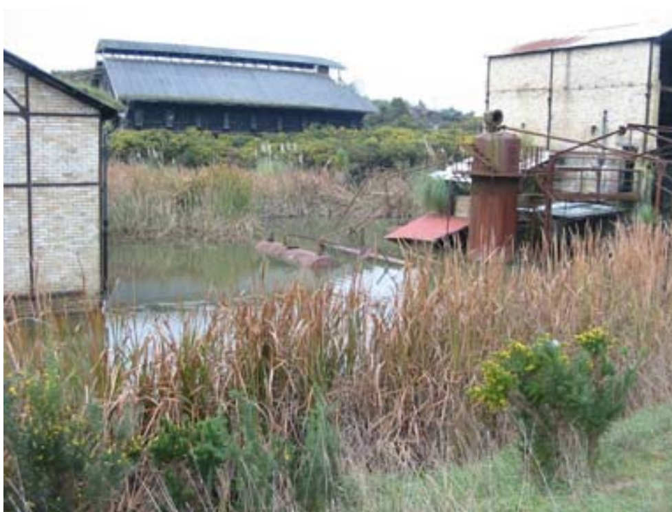
Photo 3: Flooded site looking towards the Briquette Plant and above ground storage tanks
