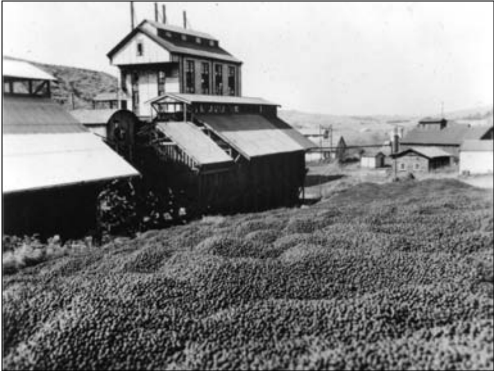
Photo 2: WCP showing the Lurgi Retort building, screening plant. Note the stored carbonettes in the foreground.
