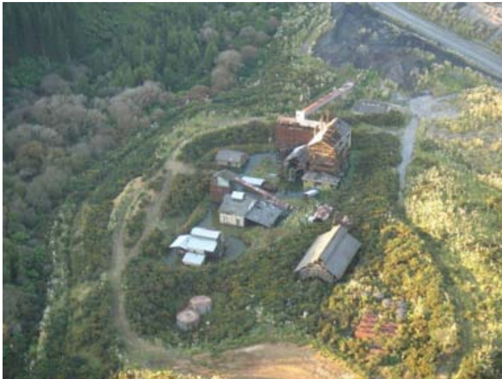
Photo 1: Waikato Carbonisation Plant (April 2007) prior to dewatering
