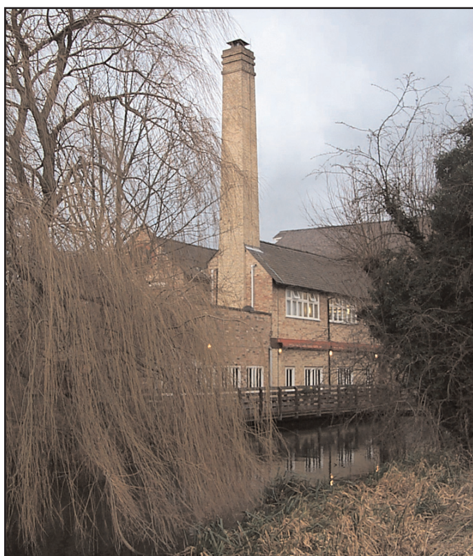
Chimney, rear of Newnham Mill
