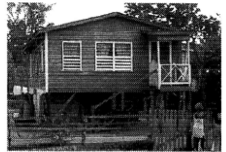
Wooden house raised off the ground to prevent flooding in case of a hurricane.
