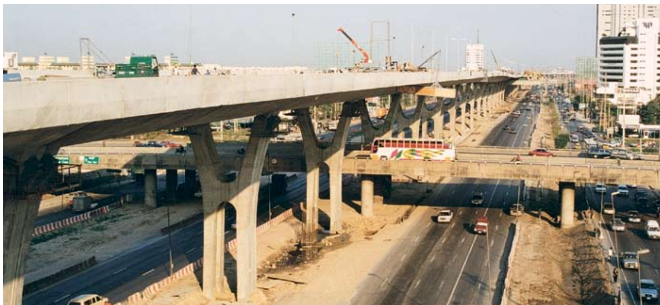
Fig. 19. The new Bang Na Expressway was completed in January 2000. This picture was taken in December 1999. Figs. 17, 18 and 19 are published through the courtesy of Jean Muller International.
