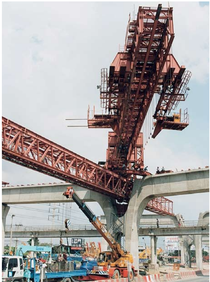
Fig. 7. Erection sequence for portal segments.
