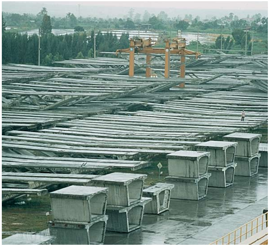
Fig. 14. Storage area for D6 and D2/D3 segments.
