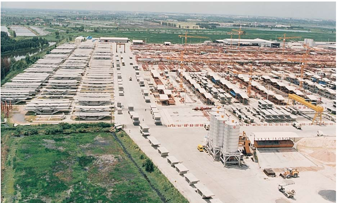
Fig. 13. Layout of precasting yard.
