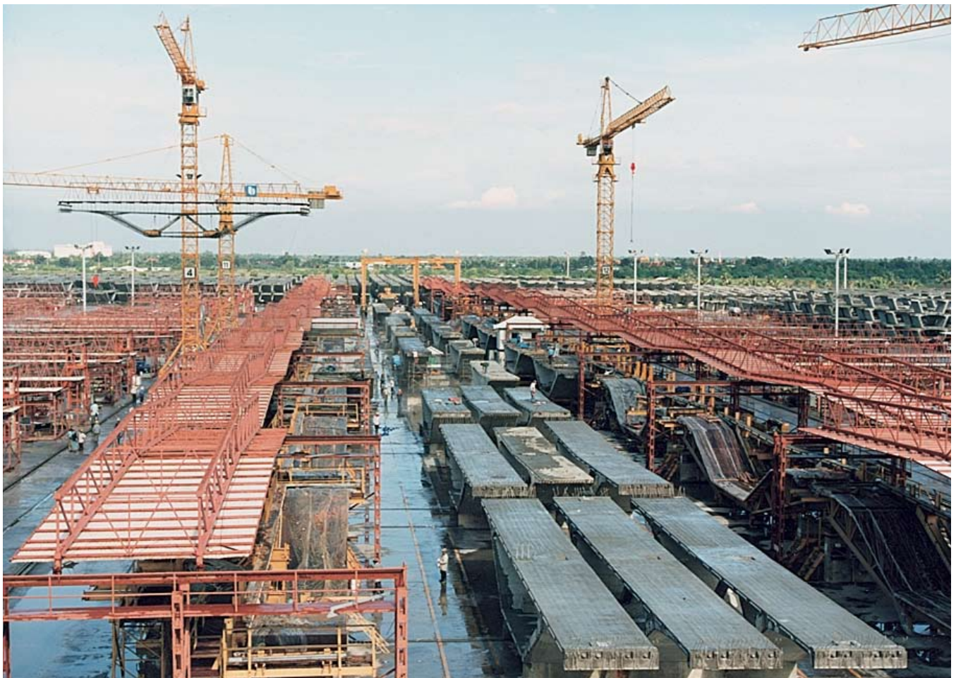
Fig. 15. D6 segment production line.
