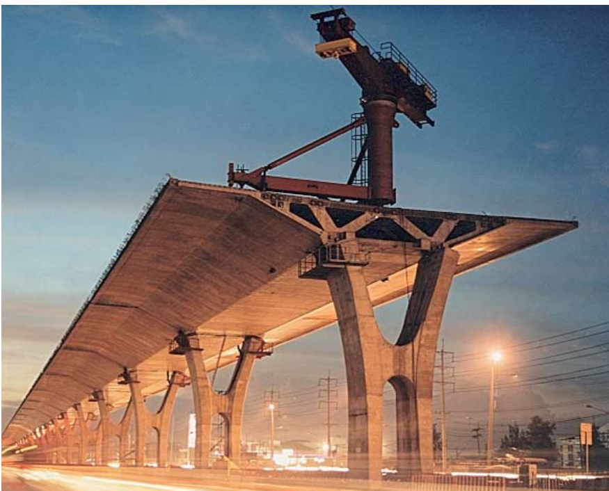
Fig. 3. Main line span of 44.40 m (146 ft).
