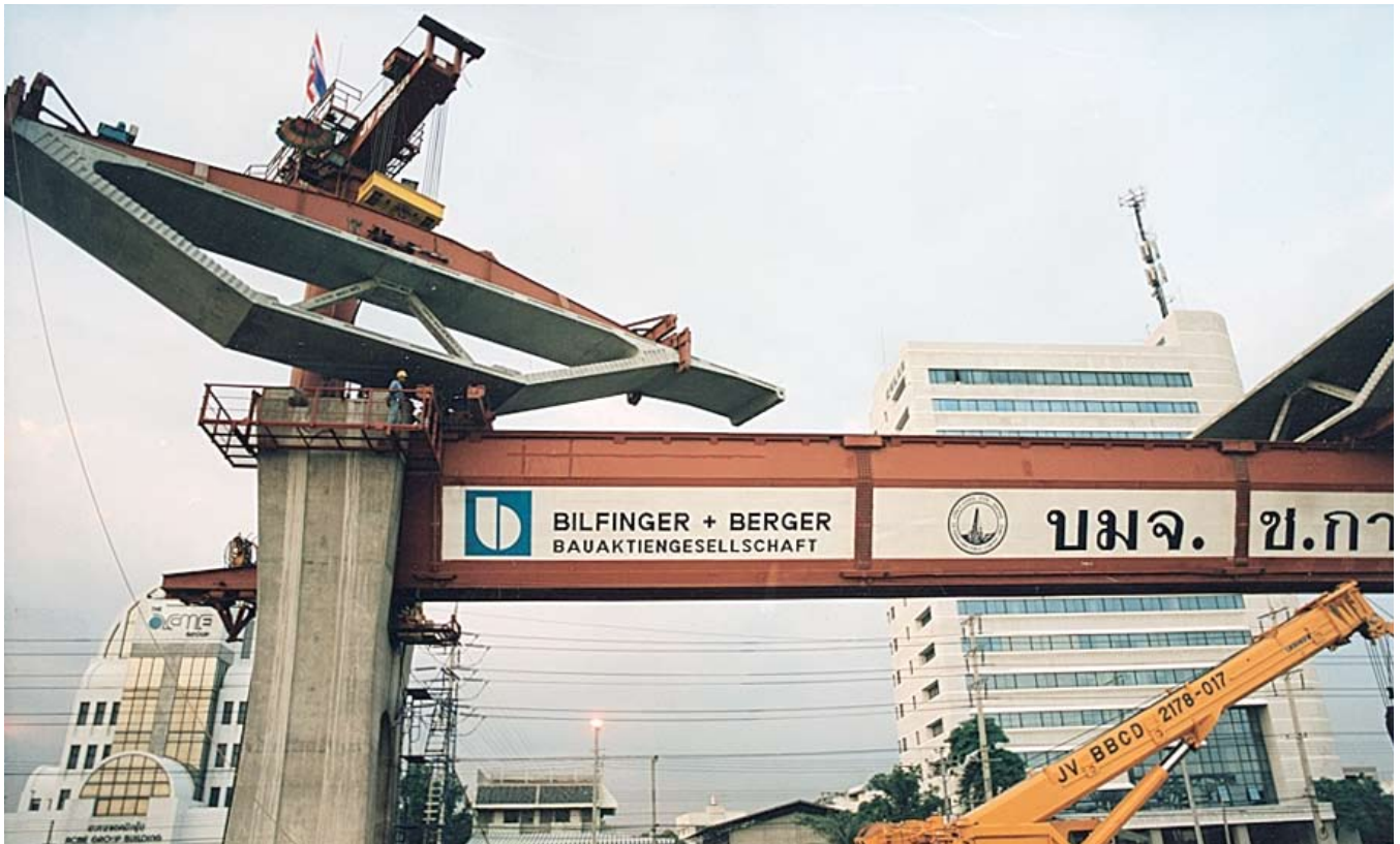
Fig. 12. Underslung erection girder.
