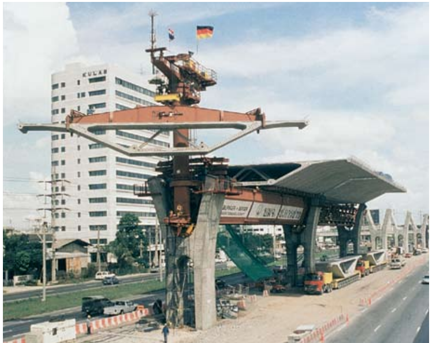
Fig. 17. Positioning of Segment D6 on mainline column.
