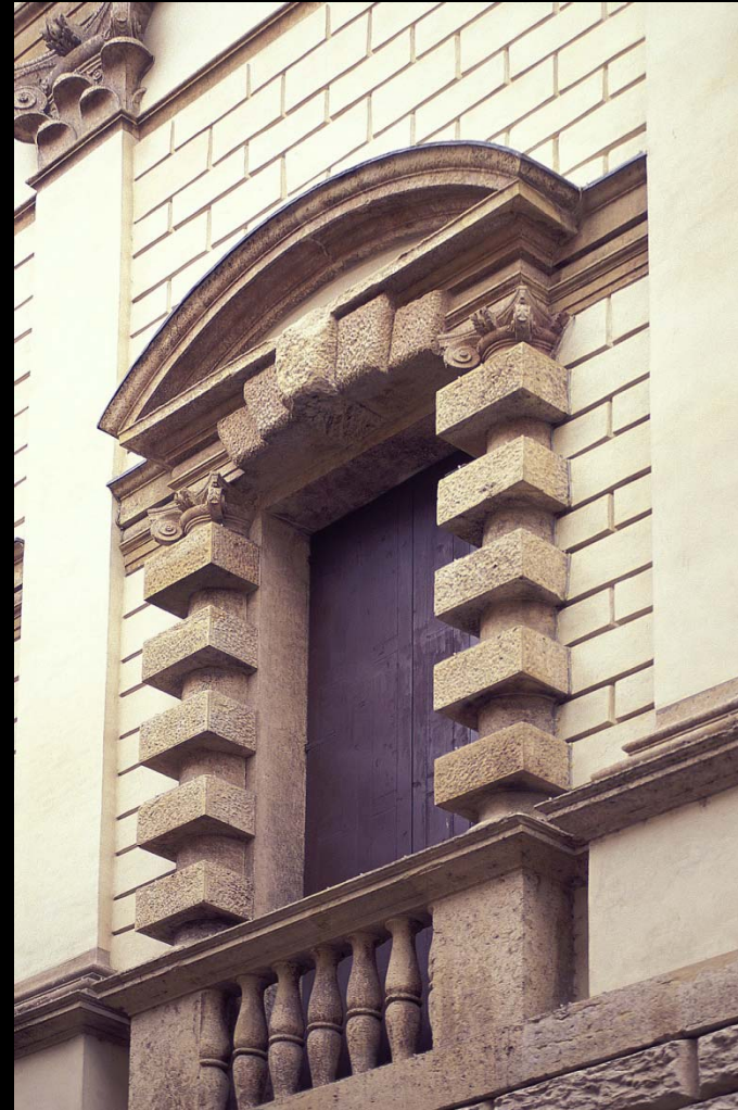
Palazzo Thiene – detail at window surround
