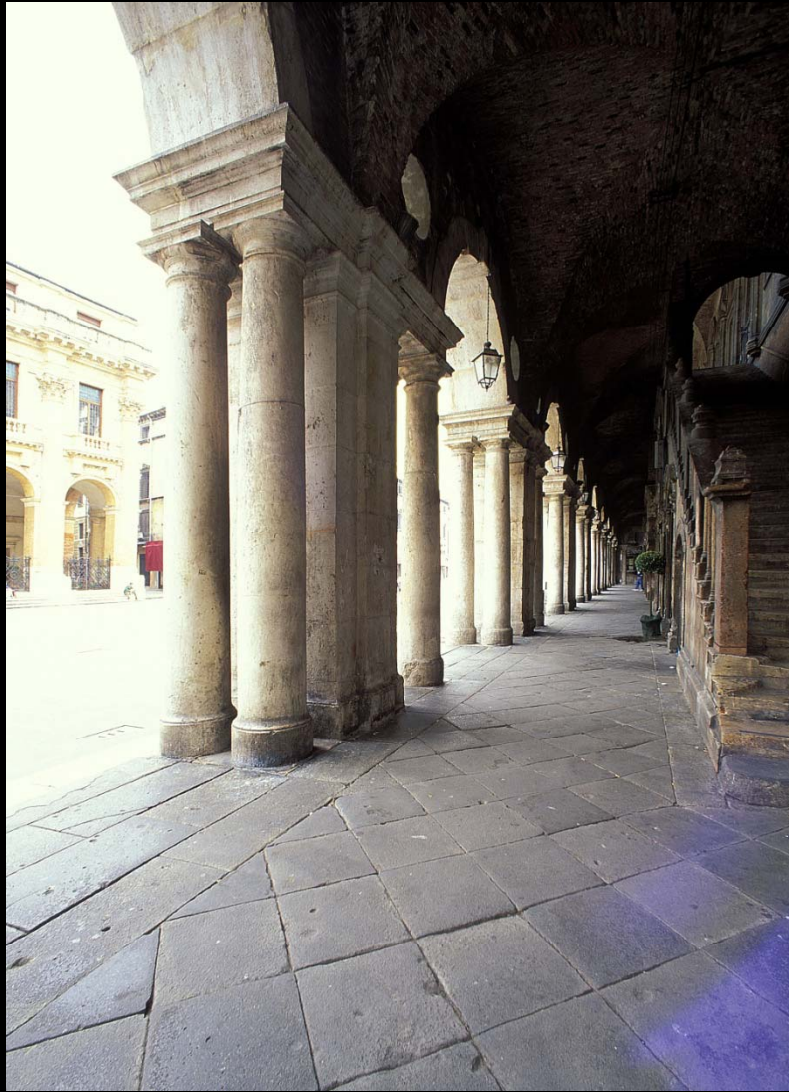
Interior view of arcade
