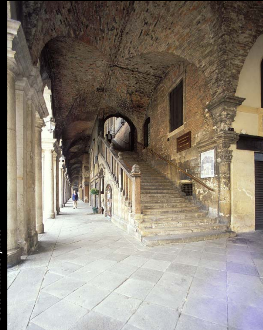
Stairs to upper level
