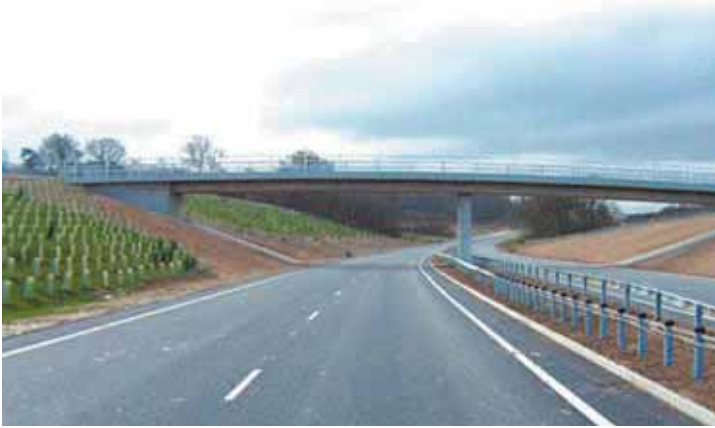
[Pierce Barn Bridge]
