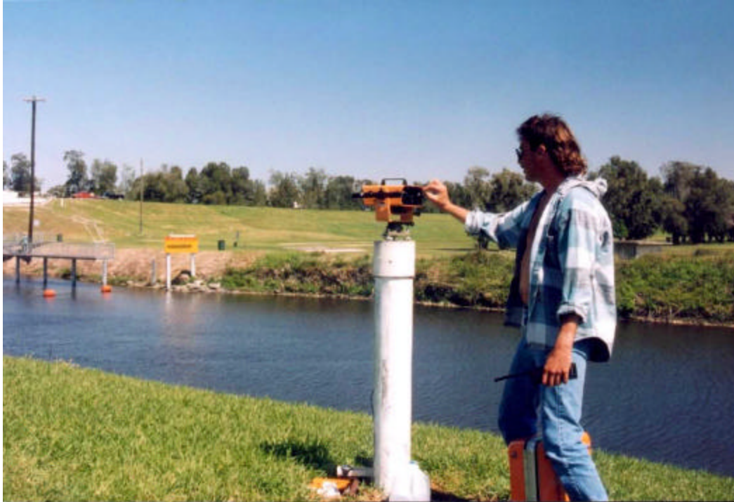
Figure 5-2. EDM observations at control structure in Central & Southern Florida Flood Control Project. EDM force-centered in concrete pedestal at external reference point. (Jacksonville District and Arc Surveying & Mapping, Inc.)
