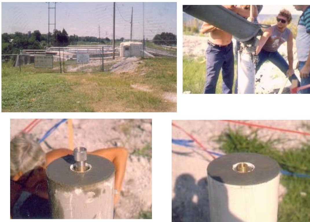
Figure 2-7. Reference point monumentation. Concrete pier construction vicinity of a hurricane gate structure. Forced centering plug set into concrete pier. (Jacksonville District)
