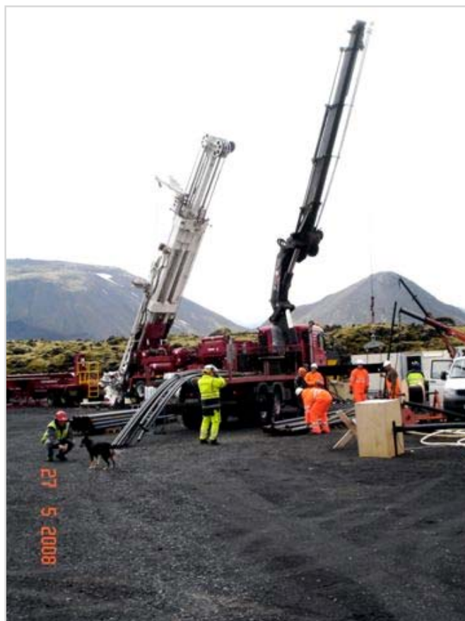
Figure 4 – Drilling of a new monitoring well HK-34 at the CO 2 injection site in May 2008. Photo: Guðmundur Lárusson.
