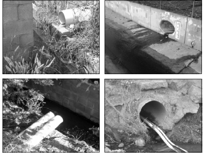
PHOTOS OF WASTEWATER DISCHARGES FROM GREENHOUSE OPERATIONS INTO CREEKS THAT DRAIN INTO CARPINTERIA SALT MARSH.
