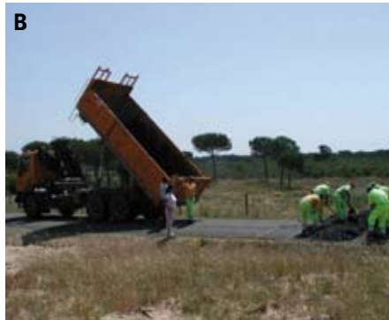
FIGURE 2. (A). FAUNA UNDERPASS PLACED IN A ROAD OF DOÑANA AREA. (B). CONSTRUCTION OF SPEED BUMPS IN A ROAD OF DOÑANA AREA.
