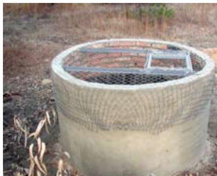
FIGURE 3. WELL COVERED WITH A METALLIC NET PROTECTED FROM THE ENTRANCE OF IBERIAN LYNXES. DROWNING IN WELLS WAS DETECTED AS A RELEVANT CAUSE OF MORTALITY DURING THE 90'S.
