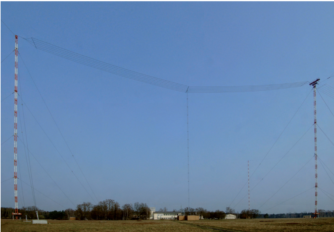
Figure 7: Transmitting radio station Mainflingen of Media Broadcast GmbH, in the foreground: antenna house 4 (made of red bricks) with DCF77 operating antenna, in the background: transmitter house 2 (white building)
