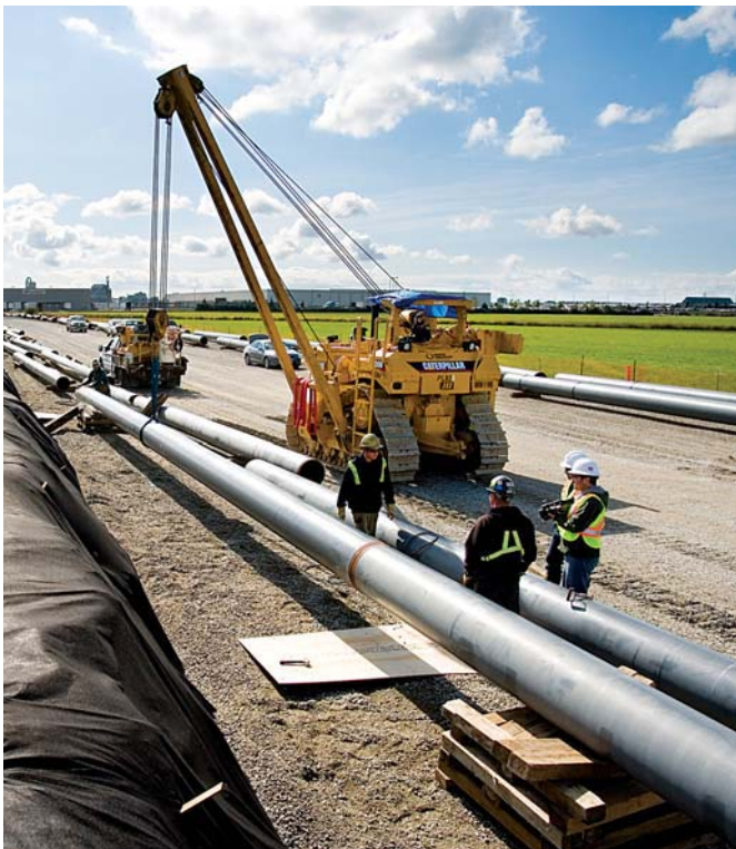
The approximate $27 million Fraser River South Bank South Arm Rehabilitation Project is expected to be in service by the end of August 2010.
