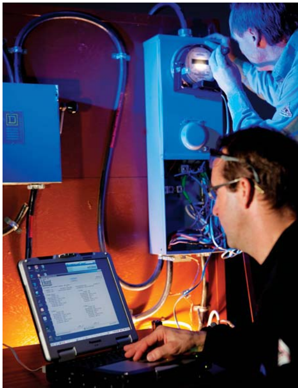
FortisAlberta's Automated Meter Infrastructure Project enables customers to better monitor and manage their energy consumption.
