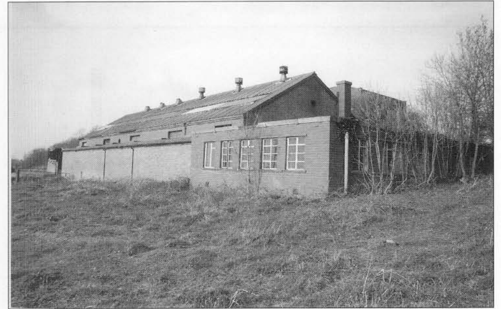
Plate 6. A now demolished 'functionalist' bath house at Pensford.
