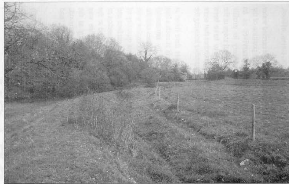
Plate 2. This earthenwork leat transported water to drive the water wheels at Vobster Colliery; the coal mine lies in the centre background of the photograph.
