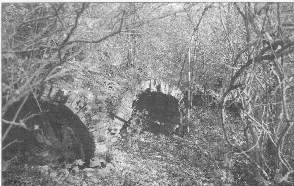
Plate 1. The nationally unique coking ovens at Vobster Breach.
