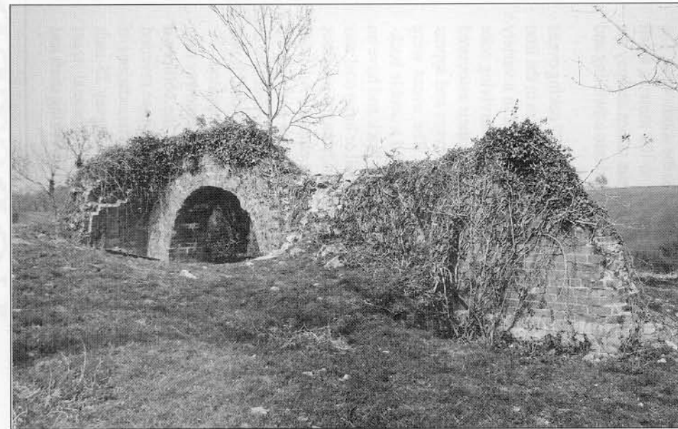
Plate 4. The Guibal fanhouse at Mackintosh replaced an earlier air furnace at the foot of the upcast shaft in the early decades of the 20th century.
