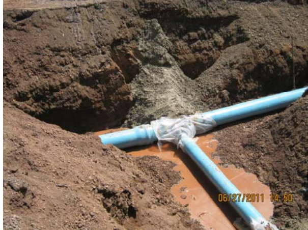
Figure 7: Watermain Tee Connection
