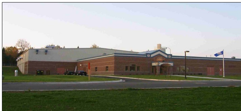
Figure 5: Moncton Water Treatment Plant
