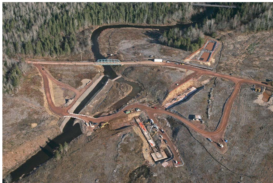
Figure 2: Aerial view of Tower Road Dam Construction Site
