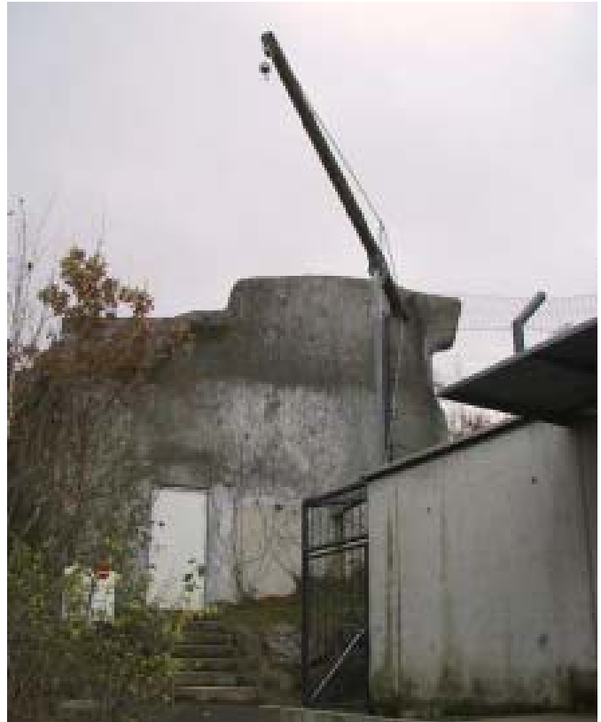
Boom - The feeding boom can be swung to the outside of the exhibit to hang meat. ©Monika Fiby, 2004
