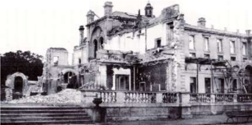
The demolition of Clumber House
