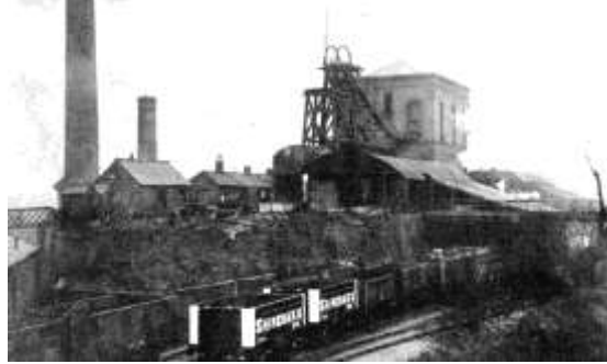
Shireoaks Colliery railway
