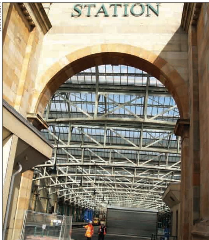
Glasgow Central High Level station's famous arch will soon have track running right through it to serve platform 12 and the brand new platform 13 as part of the Glasgow Central High Level Paisley Improvements Project.
