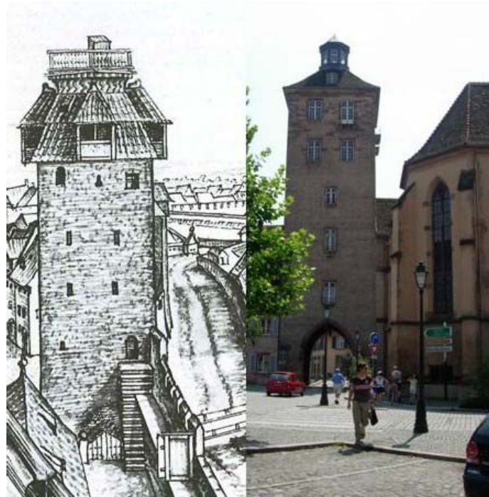
1. The top of Strasbourg Hospital Gate before its covering by the turret lantern (1671 pen-and-ink sketch by Joh. Jacob Arhardt) and nowadays (© Cabinet des Estampes , reproduced with permission, & A. Heck). The structure visible on the ancient terrace is likely a shelter.
