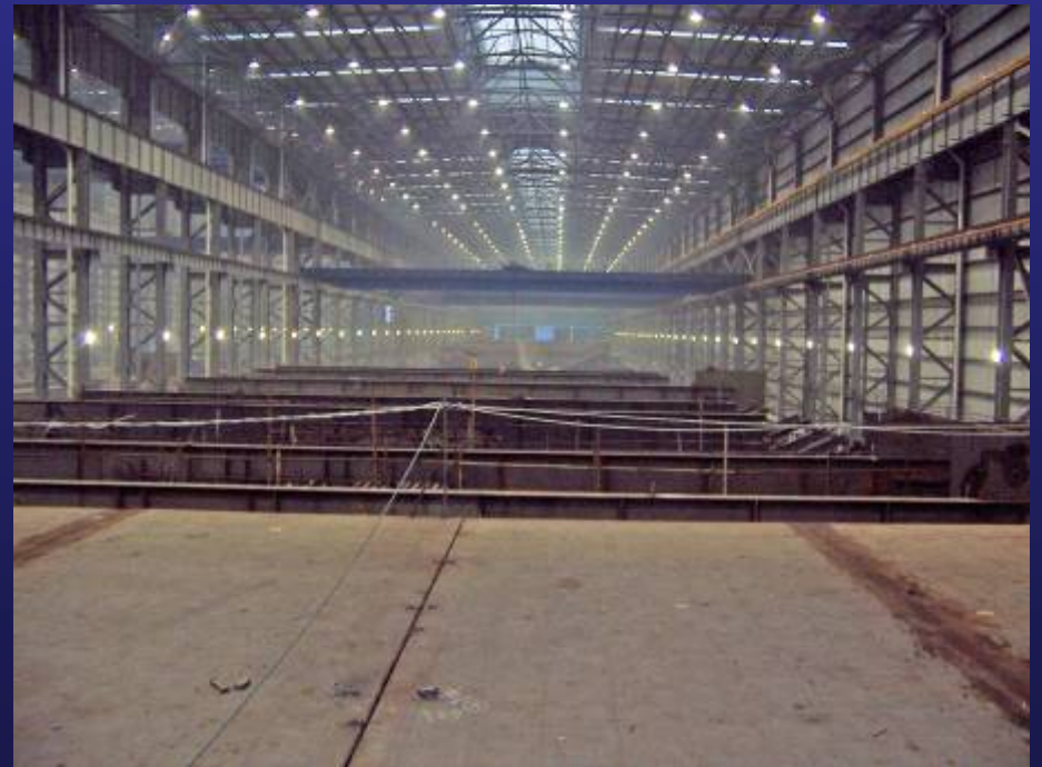
OBG Lifts Lined Up
