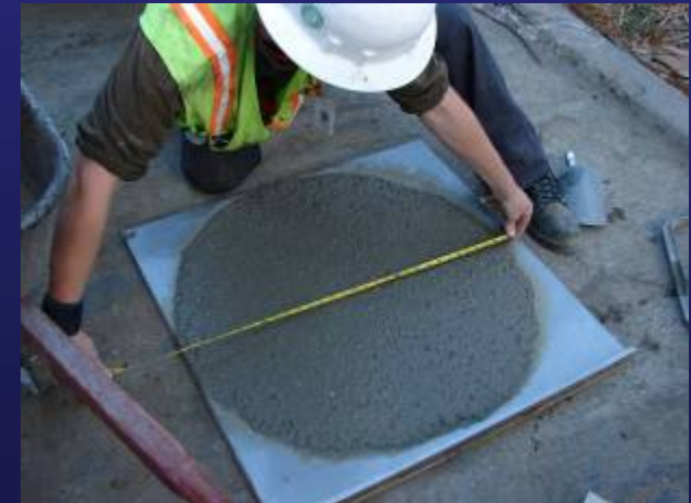
Spread Test Performed During Self Consolidating Concrete Pour Mock-up
