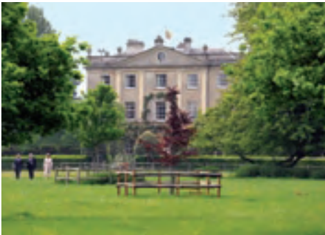
ABOVE FROM TOP TO BOTTOM Clarence House, where more efficient boilers have been installed.
