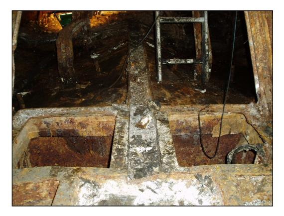
Deformation of the double bottom below the fish hold. Photograph taken in way of the bilge well.
