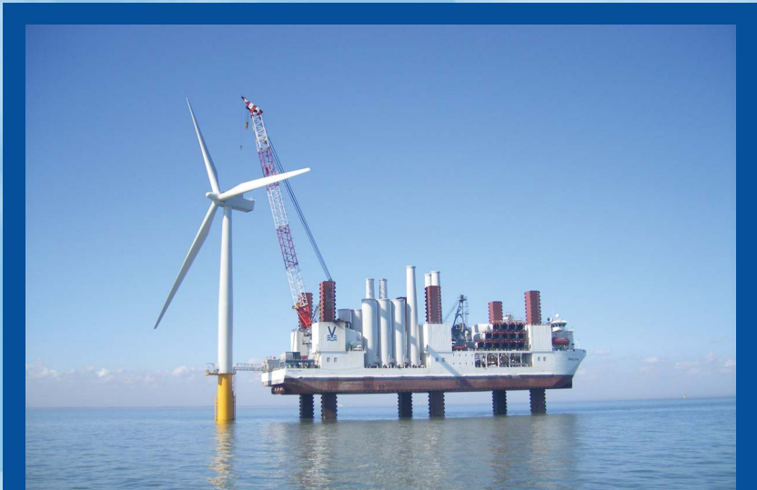
Construction of the Lynn Offshore Wind Farm, owned by Centrica
