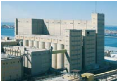
Mill and silo complex, Kuwait
