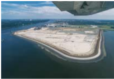
Extension for Airbus production area, Hamburg, Germany Construction supervision
