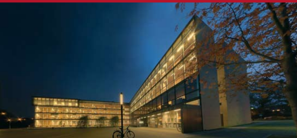
University Library in Rostock, Technical building equipment
