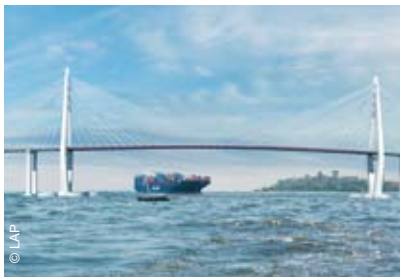
Southern Karachi bypass "Karachi Harbour Crossing", Pakistan, together with LAP
