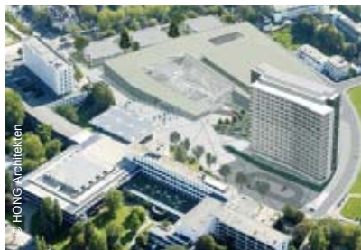
World Conference Center, Bonn, Germany Technical building services and equipment
