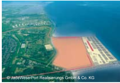
Deep water harbour, Wilhelmshaven, Germany Design, construction supervision
