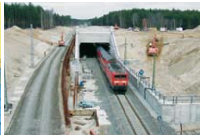
Tunnelling under the Havel-Oder waterway, Germany
