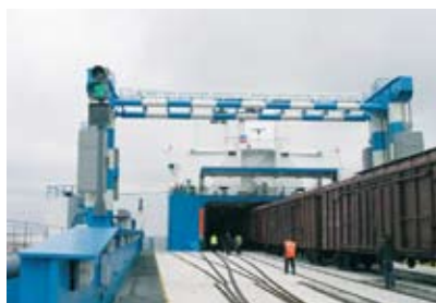
Railway and Ro-Ro ferry terminals, Ust-Luga and Baltiysk, Russian Federation
