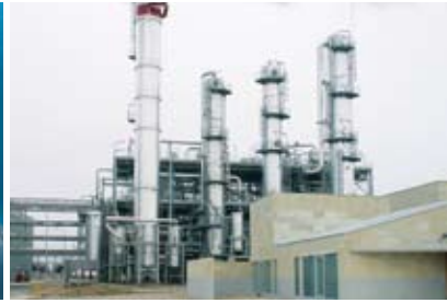
Construction of a bio-ethanol plant, Germany
