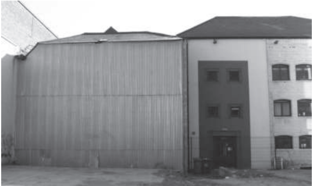
Warehouse at 42 Waring Street
