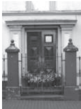
Gracehill Old School, Church Road (before restoration)
