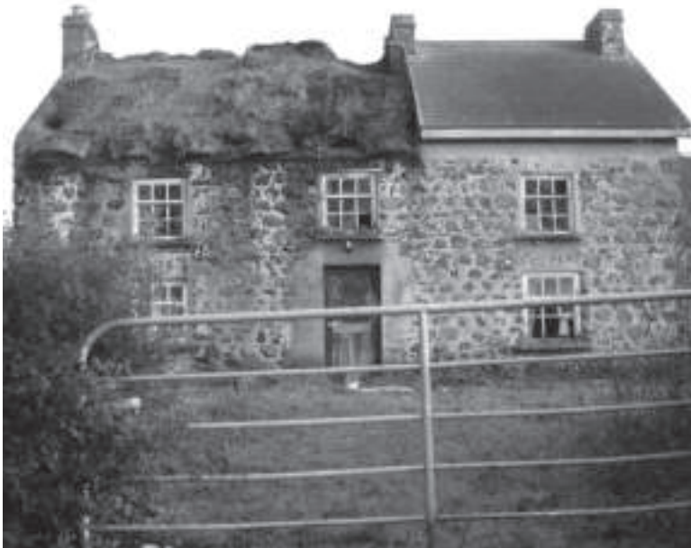
20 Scroggy Road, Glenavy (before restoration)
