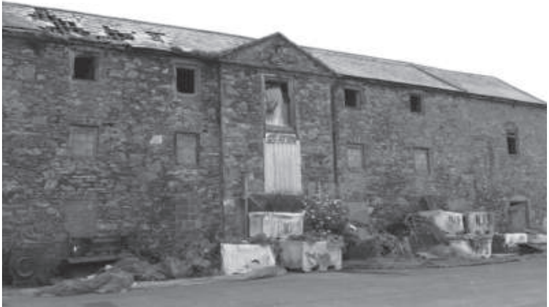
Harbour Warehouse, North Quay, Ardglass
