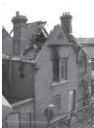
Fire Station, Hawkin Street, Derry (before restoration)
