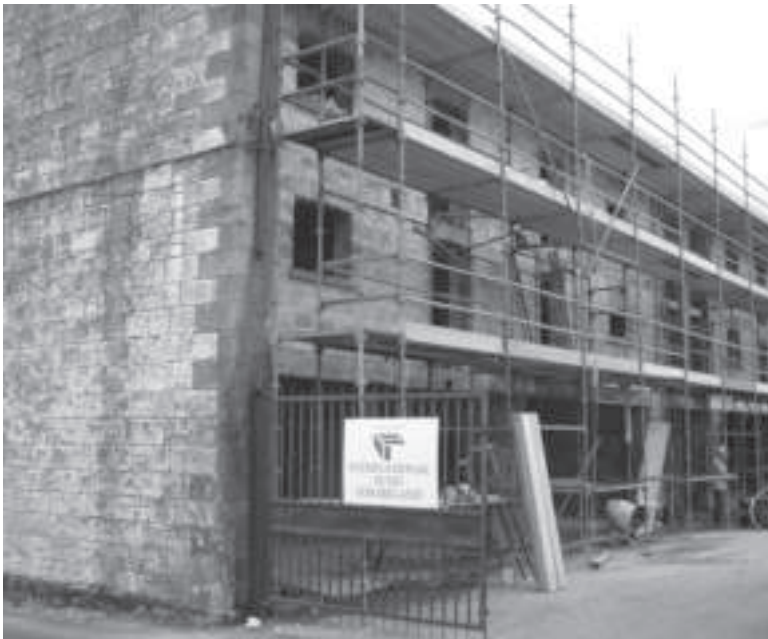
Corn Stores, Market Street, Moneymore (during restoration)
