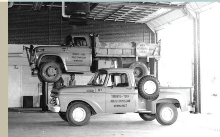
Toronto and York Roads Commission Garage
