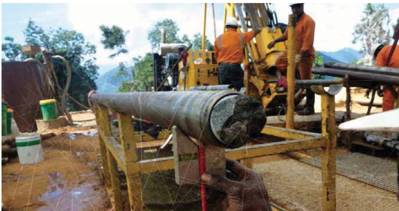
Kurunga prospect drilling operations
