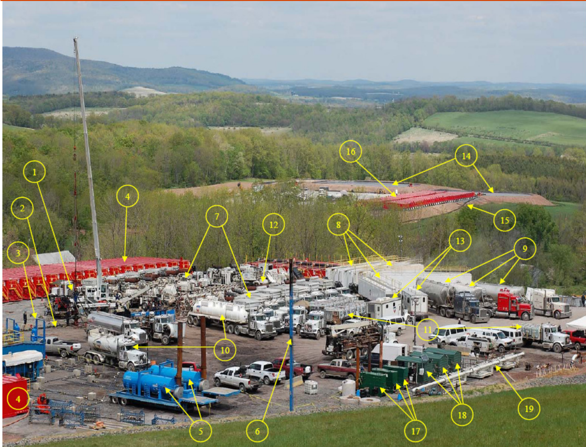
Figure 2.5: A well site during a single hydraulic fracturing operation (New York State, 2009)
