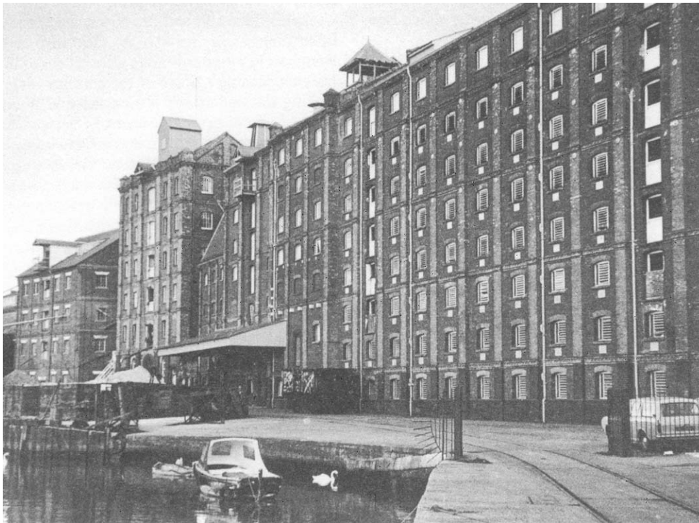
Plate IX The massive eight-storey, seventeen-bay malting at Mistley, Essex. Erected in 1896–7 by the firm of Free, Rodwell and Co. the Grade II listed building incorporated many important technological innovations.
