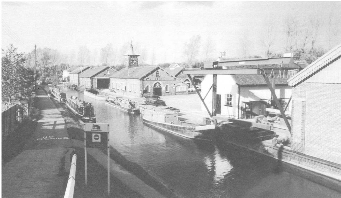
Plate X Bulbourne canal works and boat lift at Tring, Hertfordshire. Copyright: Hertfordshire County Council
