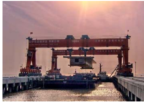
Fig. 22 Box Girder Onto Ship
