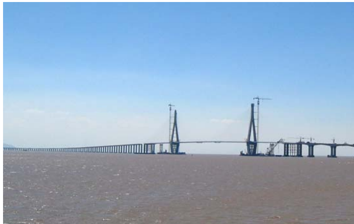
Fig. 16 Main Navigation Spans of the Jintang Bridge
