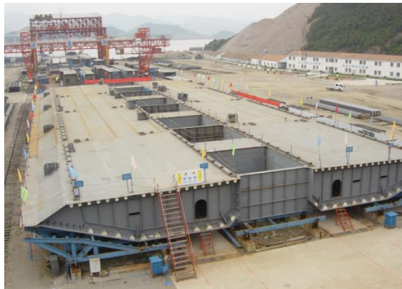
Fig. 11 Structure of Steel Box Girder
