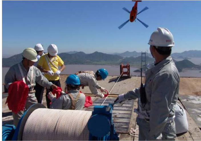
Fig.14 Towing Pilot Cable Across Sea by Helicopter
