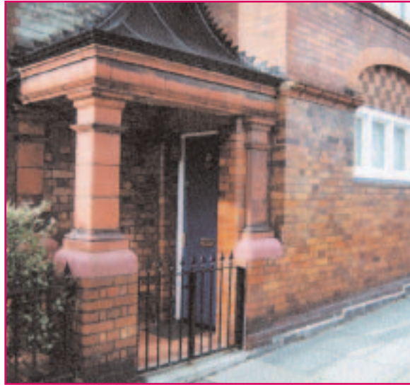
Corner treatment showing fine terracotta chequer detailing, lead canopy and reinstated railings.
