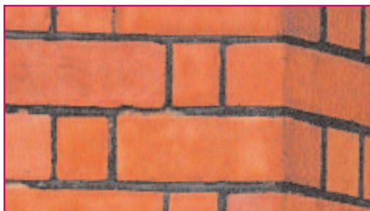
Good original pointing
