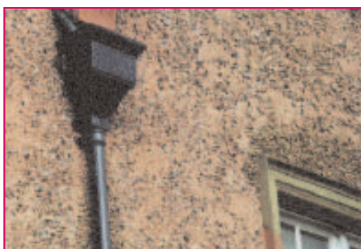
Original cast iron hopper and downpipe
