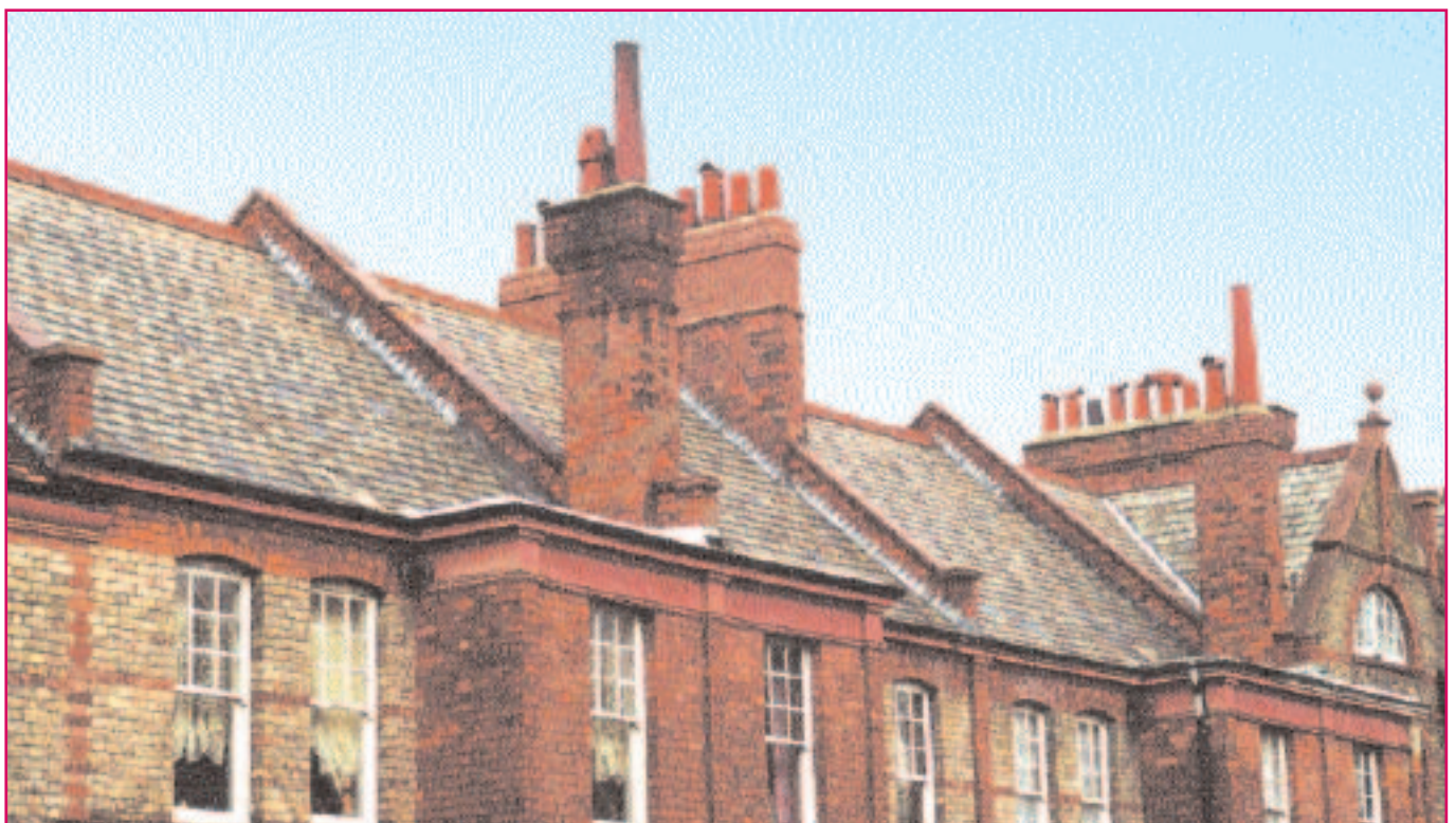
Fine weathered green slate roofing - possibly Westmoreland slates.
