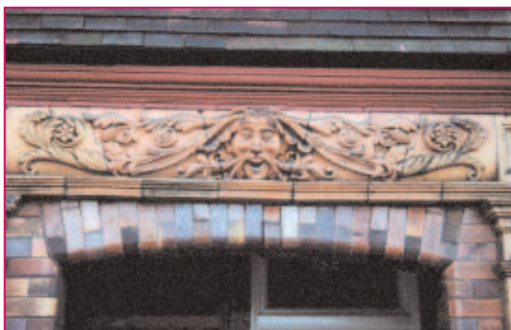
Terracotta door canopy detail.
