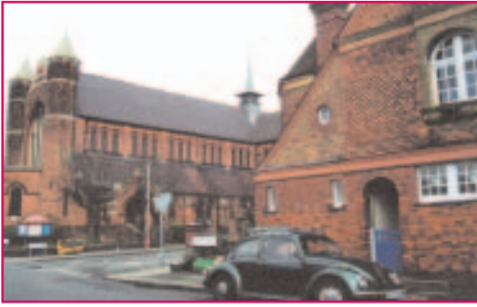
Matching materials: St. Margaret's church. In foreground matching orange brick tile-hung gable. Note coarse-rendered niche.
