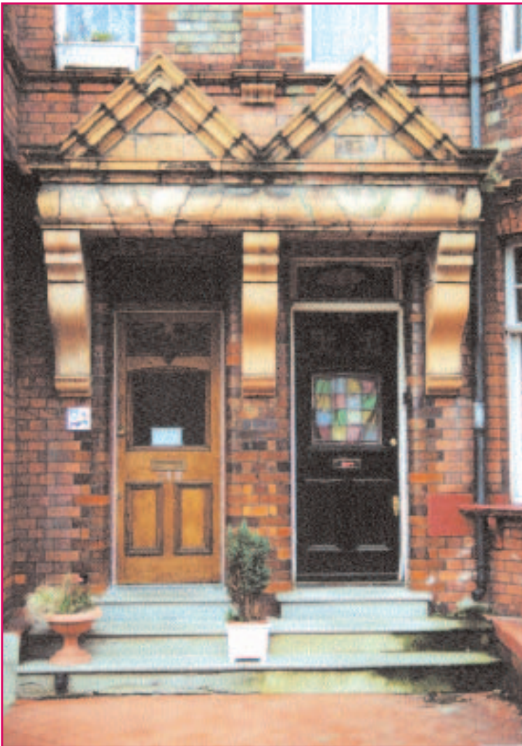
A pair of doorways with terracotta canopies and coloured glass. Note the diamond tiled forecourt.
