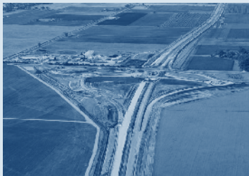
An aerial view of the Curtis Road Interchange, part of the Northern Expressway Project.
