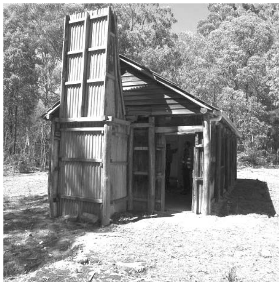
Wilson's hut: repaired timber posts and chimney
