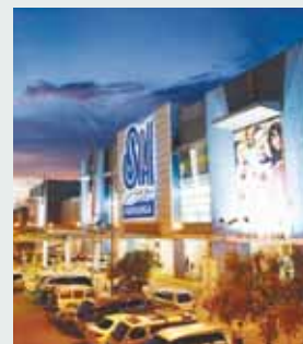
SM CITY PAMPANGA Brgy. San Jose City of San Fernando, Pampanga Year/Month Opened: 2000 November GFA: 129,102 sqm
