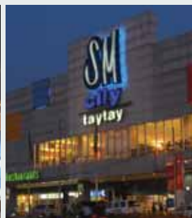
SM CITY TAYTAY Manila East Road, Brgy. Dolores Taytay, Rizal Year/Month Opened: 2007 November GFA: 91,920.16 sqm
