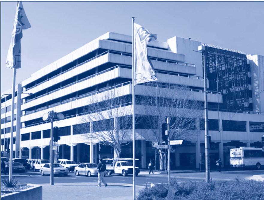
The Department's central offices at 111 Alinga Street and 62 Northbourne Avenue (Photo DOTARS)
